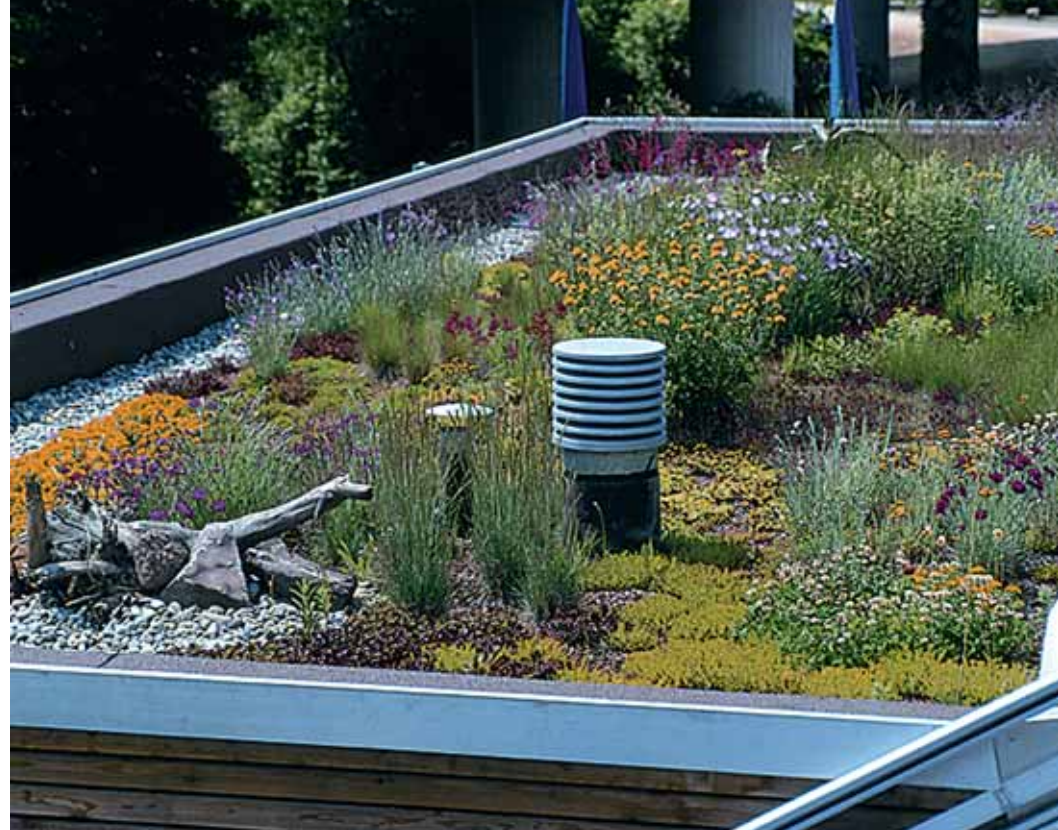
This living roof has been designed to incorporate many different habitats. ZinCo GmbH
